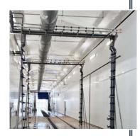
InterClean Fleet Wash systems come standard with a two-step, three manifold detergent arch. This ensures a highly effective clean by precisely targeting the detergent application over multiple areas of the vehicle.
